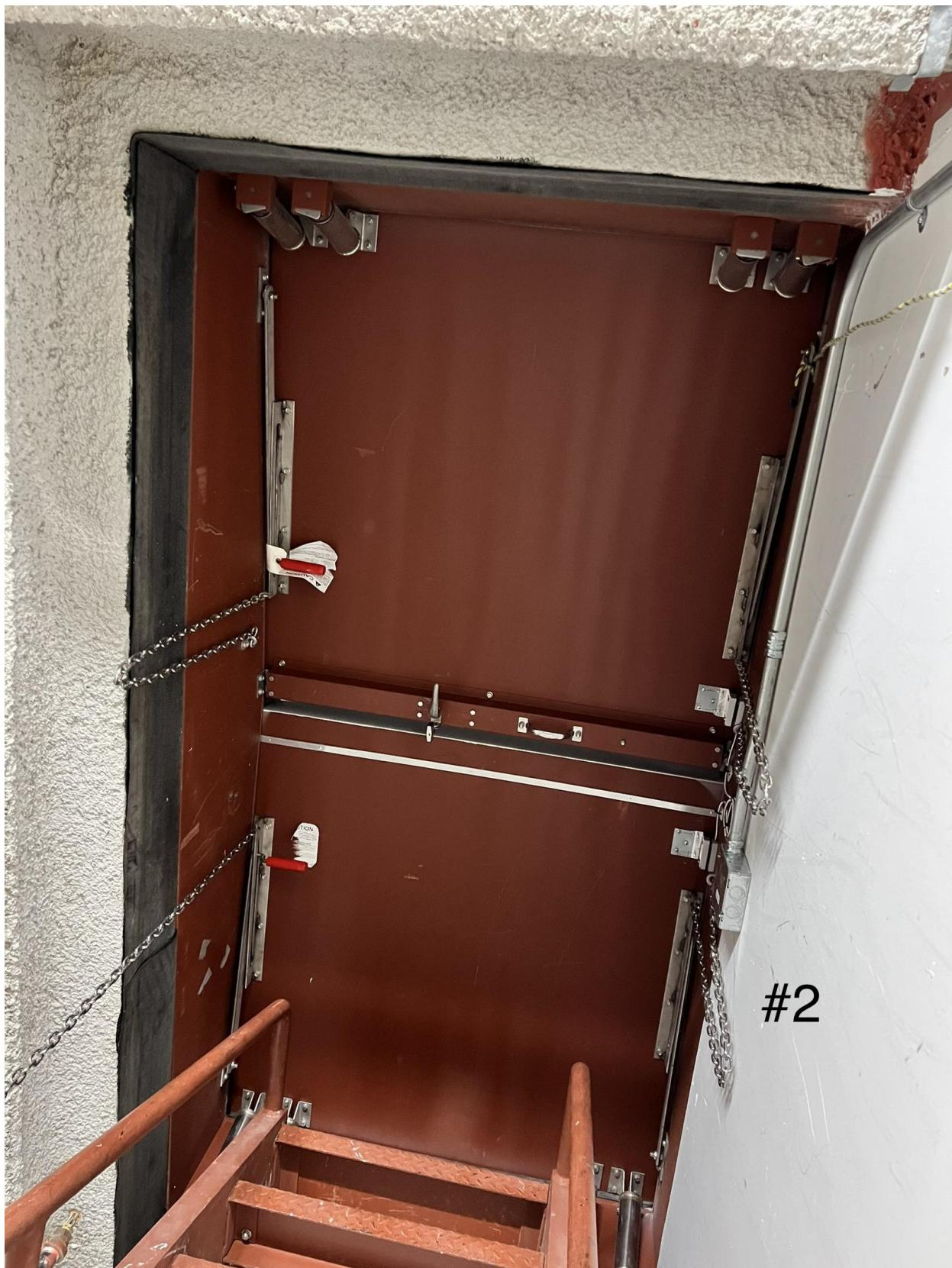
After the left door is open, you can then push open the door to the right. The right door at the top of the ladder does not open to the side to allow for reasonable egress. But rather, it opens directly in front of you in a 90 degree angle acting as a wall blocking any means of egress (Photo #3).
